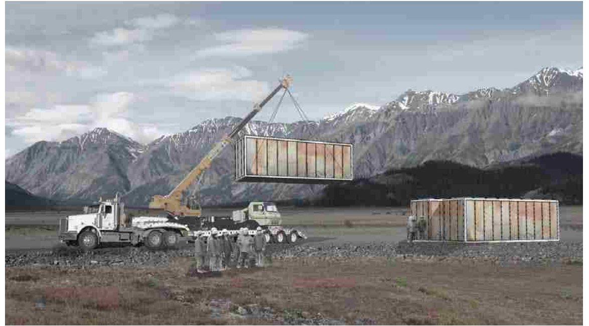
Fig: 8.19 Gallery Constructed on Site
