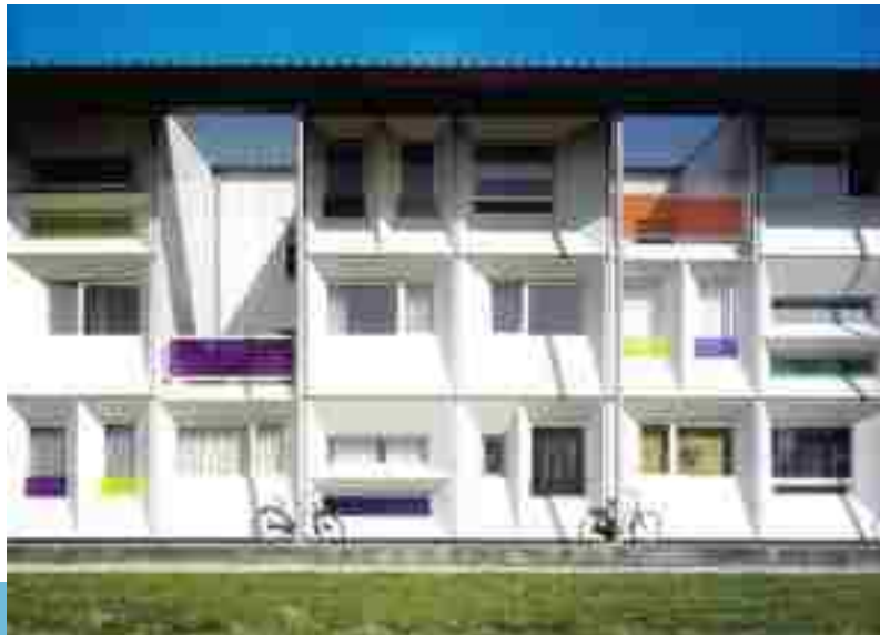
Fig: 4.6 Application of Building Container System
